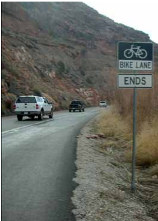
S.R. 128 has narrow traffic lanes, poor visibility, and no shoulders.
