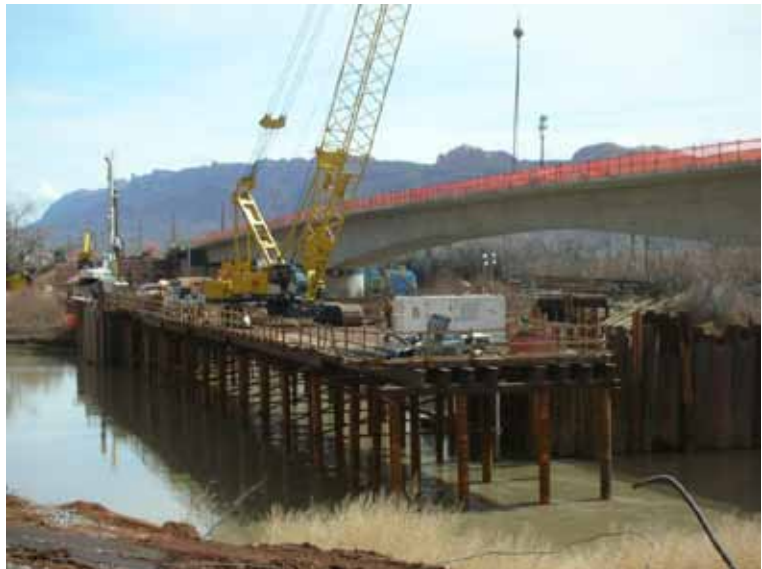
UDOT is completing a bridge section over the Colorado River.
