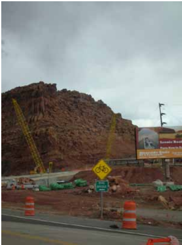
The bridge over the Colorado River will make bike travel safer.
