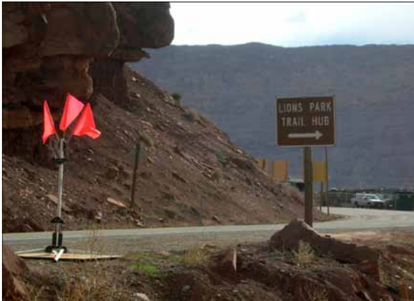
The Lions Park Trail and Transit Hub will include a park, trail, and transit hub.
